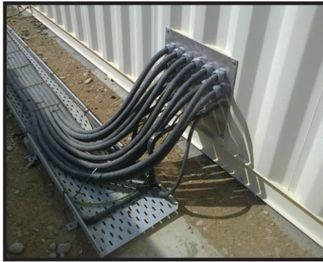
CABLE TRAY WORK
