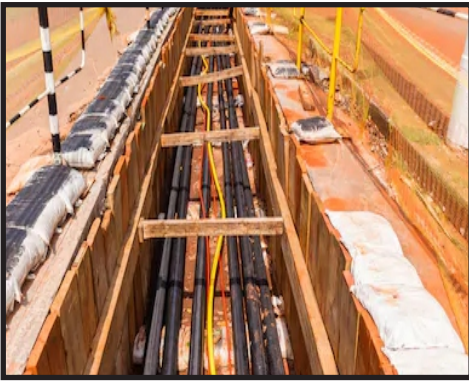
CABLE TRENCH WORK
