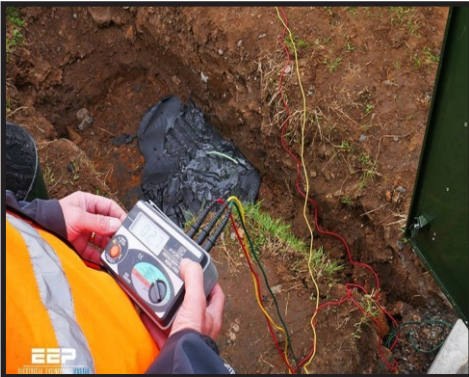
EARTHING TESTING WORK
