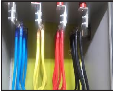
CABEL TERMINATION WORK
