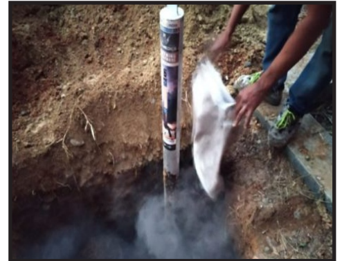
BORE EARTHING WORK
