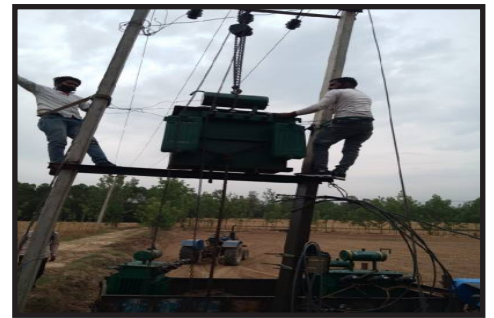
TRANSFORMER INSTALLATIONS
