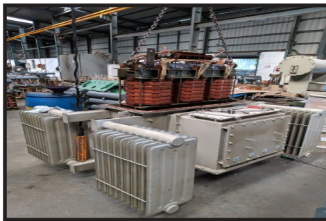
IN HOUSE TRANSFORMER MAINTENANCE
