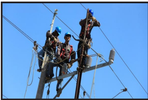
OVER HEAD LINE WORK
