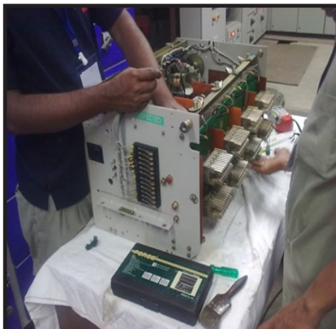
ACB SERVICING WORK
