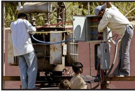
ON SITE TRANSFORMER MAINTENANCE
