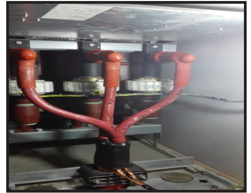
CABLE JOINTING WORK
