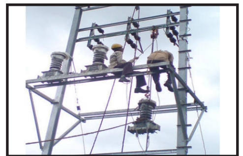
TWO POL STRUCTURE WORK
